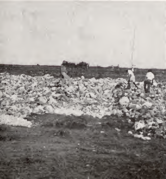
Grading the airport in Barbados
